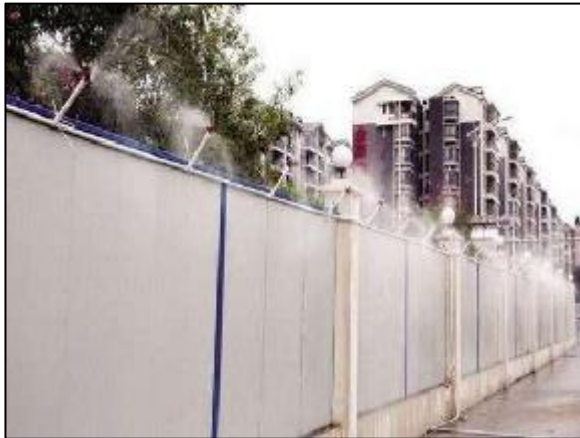
Construction enclosure and sprinkler
