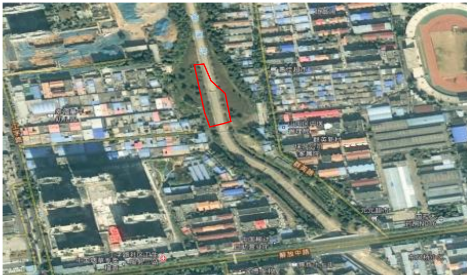
Construction camp of JZTJ105-Wengjian River Restoration
