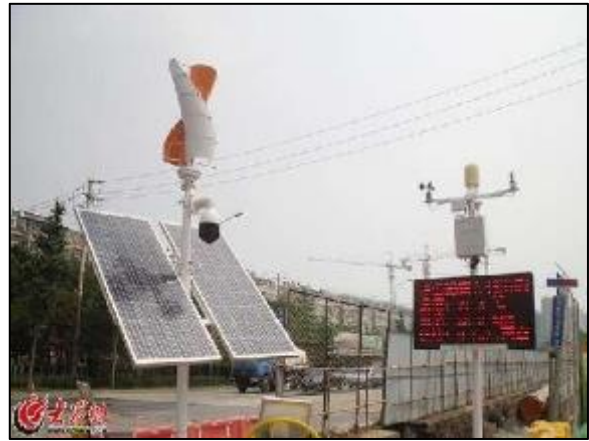
On-site monitoring and monitoring system
