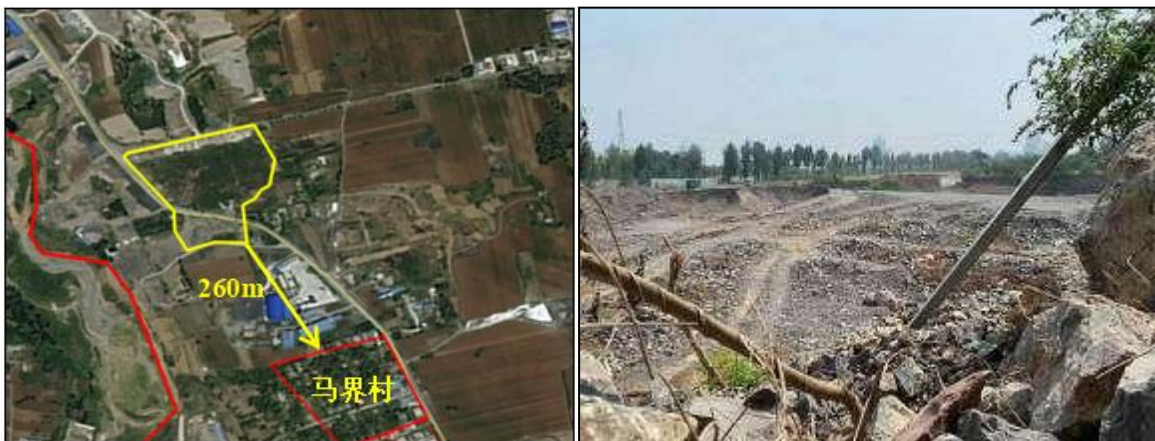
Figure G4 Location and status of spoil ground north of Majie Village (3)
