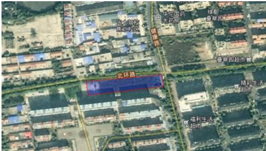
Construction camp of JZTJ112North Ring Road (Puji Road-Tabei Road) Restoration
