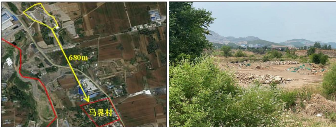
Figure G3 Location and status of spoil ground north of Majie Village (2)
