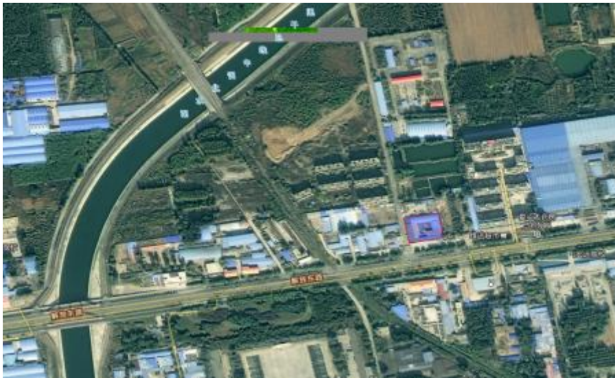
Construction camp of JZTJ120-Jiefang East Road Restoration
