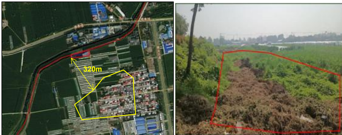
Figure G8 Location and status of spoil ground in Xinzhuang Village (7)
