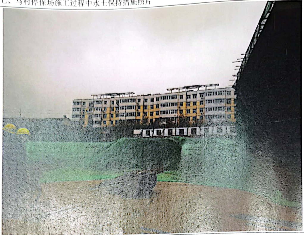
扰动面临时苫盖
